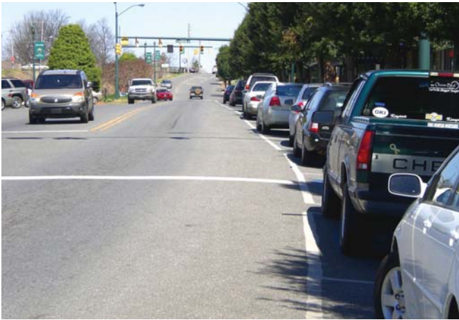
Battleground Avenue parallel on-street parking
