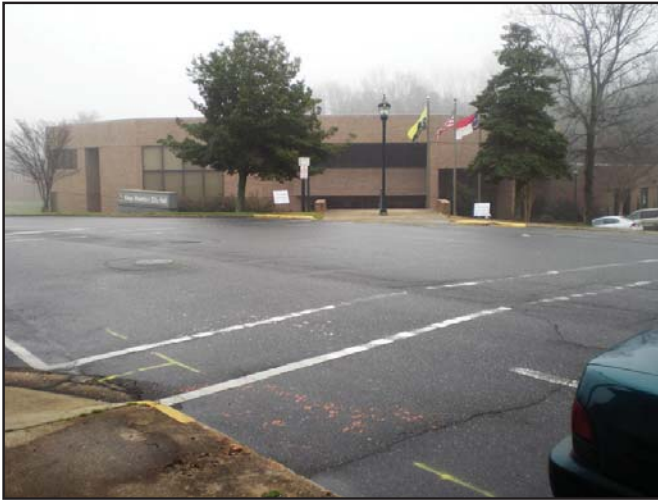
Faded crosswalk at intersection of Cherokee & Gold Streets
