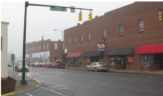
Downtown 2 story buildings on Gold Street with vertical mixed-use potential
