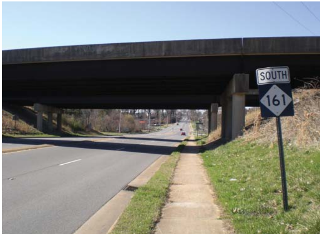
Cleveland Avenue crossing under US 74 Bypass
