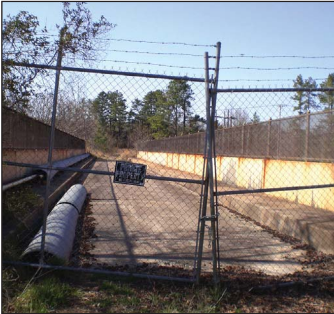
Mining Bridge over I-85
