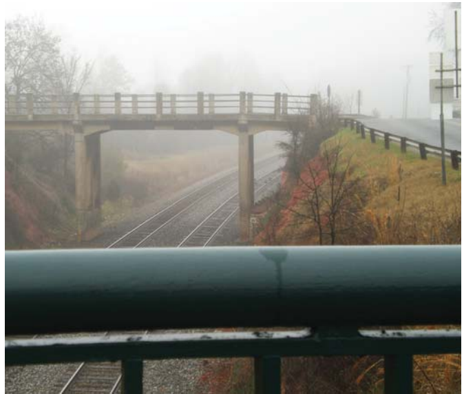
South Railway Bridge viewed from King Street Bridge
